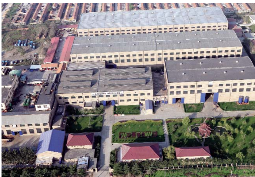
Aalborg Industries' marine boiler and heat exchanger factory in Jiaozhou near Qingdao, China.
