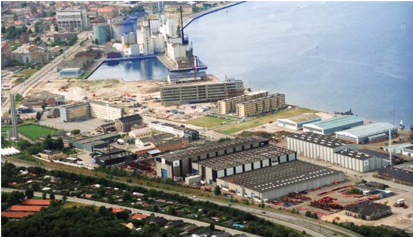
Aalborg Industries' corporate headquarters, heat exchanger business centre and factory in Denmark.
